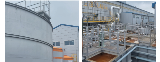
The new wastewater treatment center at SeAH Coated Metal
